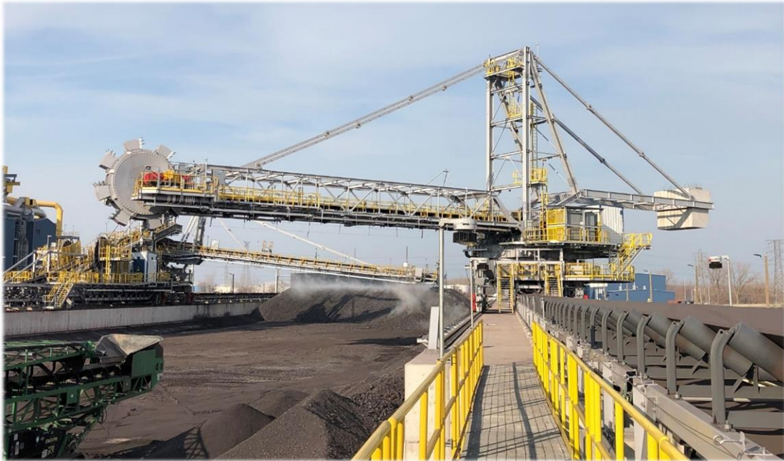
TAKRAF bucket-wheel reclaimer for handling HBI in the US can be seen in the foreground with stacker behind.
