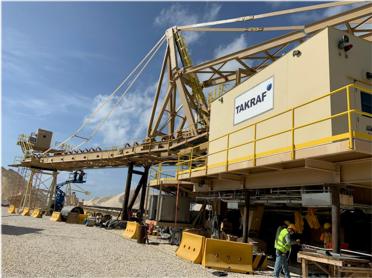
Site erection of the 6,000 t/h TAKRAF stacker in Mexico.
