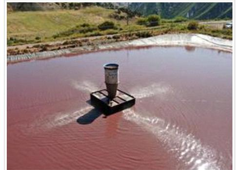
RWI Enhanced Evaporation's PittBoss(TM) efficiently evaporates viscous fluids so the remaining solids can be safely disposed of in a landfill. Its downdraft fan design does this without putting solid particles in the air and without nozzles that must be cleaned.
