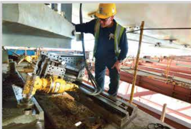
MILLING BRIDGE SHEAR KEY BASEPLATES
