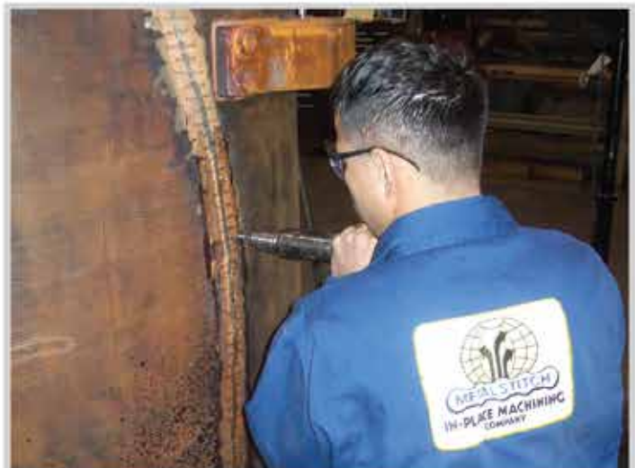
METALSTITCH® COLD CAST IRON REPAIR
